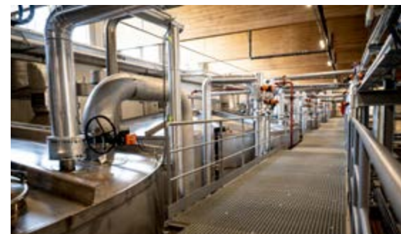
Thermal insulation of the heating system.
